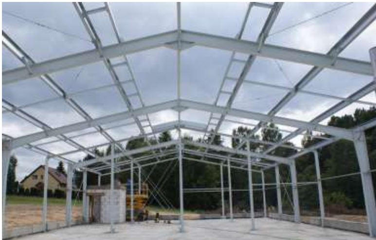
Frame construction of the hall
